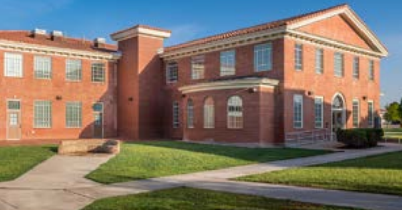
NMSBVI Alamogordo NM, Ditzler and Old WES Renovations
