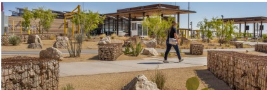
Columbus U.S. Land Port of Entry | 2020 Low Impact Design for New Border Crossing Campus. LEED Platinum and Sustainable SITES Silver Certified $1,900,000
